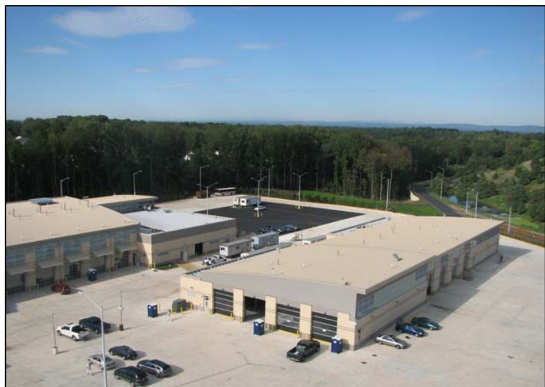
The new West Ox Bus Operations Center commenced operations on June 29, 2009.
